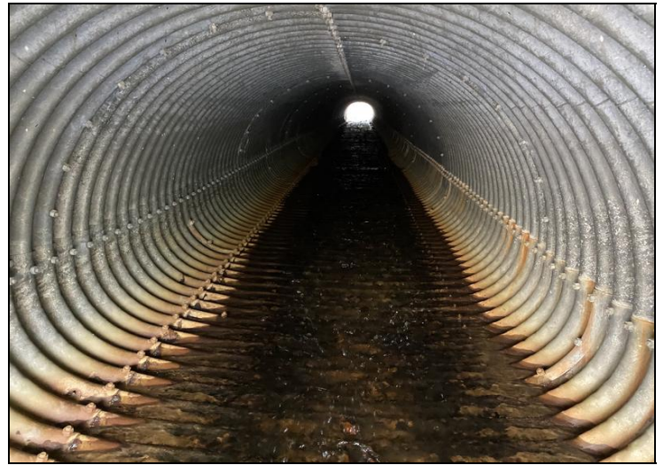
Culvert from Downstream End looking Upstream
