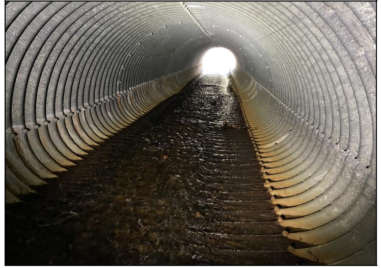
Culvert Looking Downstream from Below Roadway
