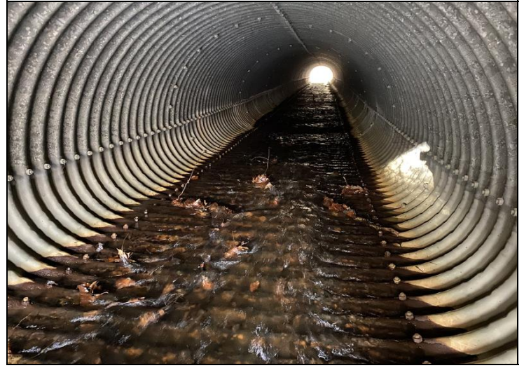
Culvert looking Downstream
