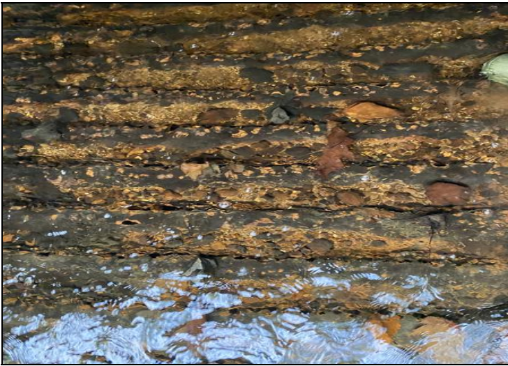
Culvert Invert at Downstream End
